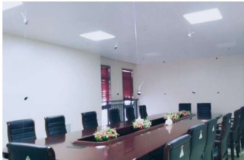
复合式空气载能辐射空调（顶板+侧墙）应用于韶山办公楼 Composite ACERS (Ceiling + Side wall) in Shaoshan
