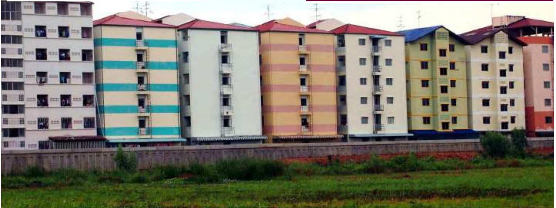
Affordable factory workers housing, but a planner's nightmare
