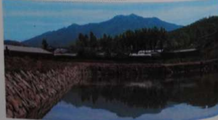
Village stream: repaired with stone embankments.
