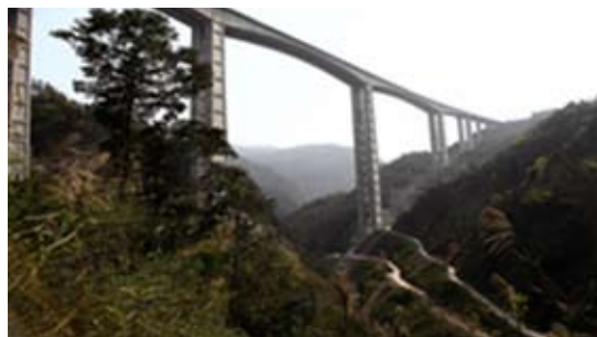
Steel tube concrete composite bridge pier 钢管混凝土组合桥墩
