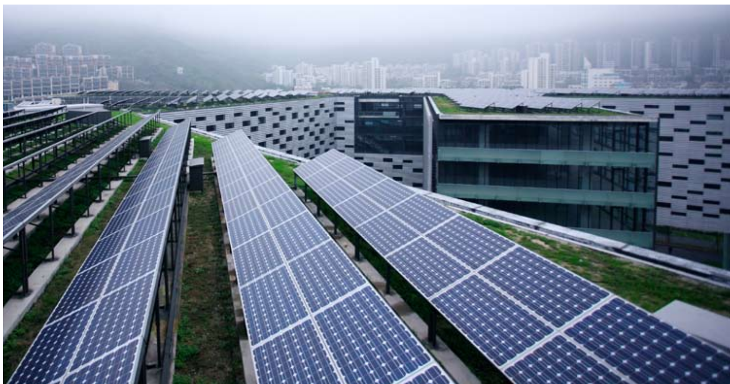
Integrated Photovoltaic System 太阳能光伏发电系统
