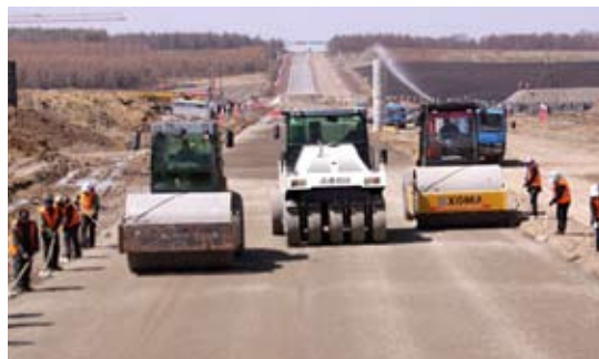
Laying crushed stone base 摊铺机轧碎石基层
