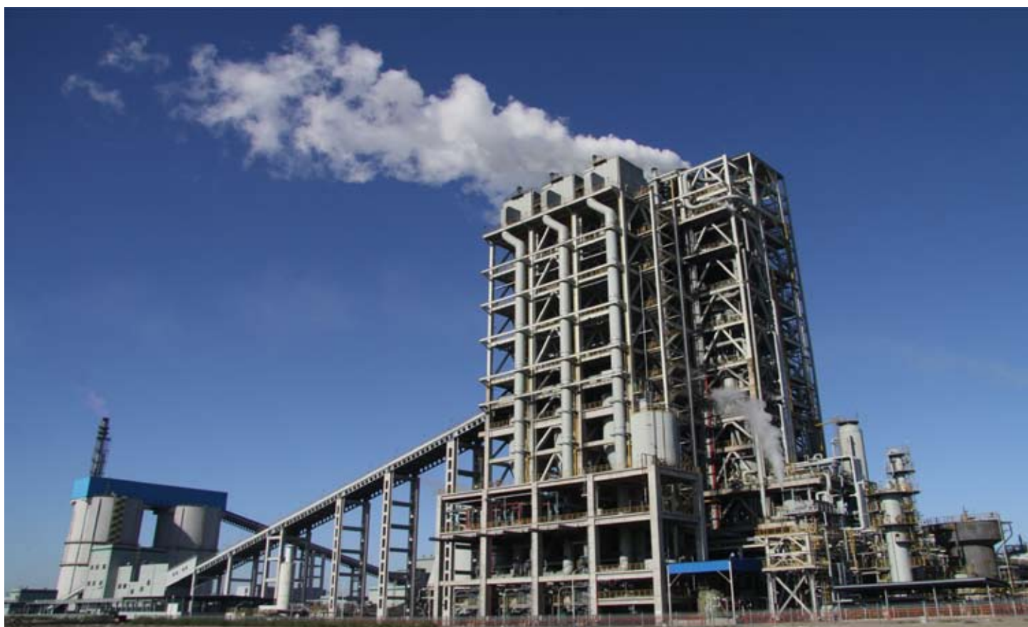
Air separation unit and gasifier 两段式干煤粉气化炉
