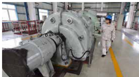
Waste Heat Generating Unit 蒸汽余热发电机组
