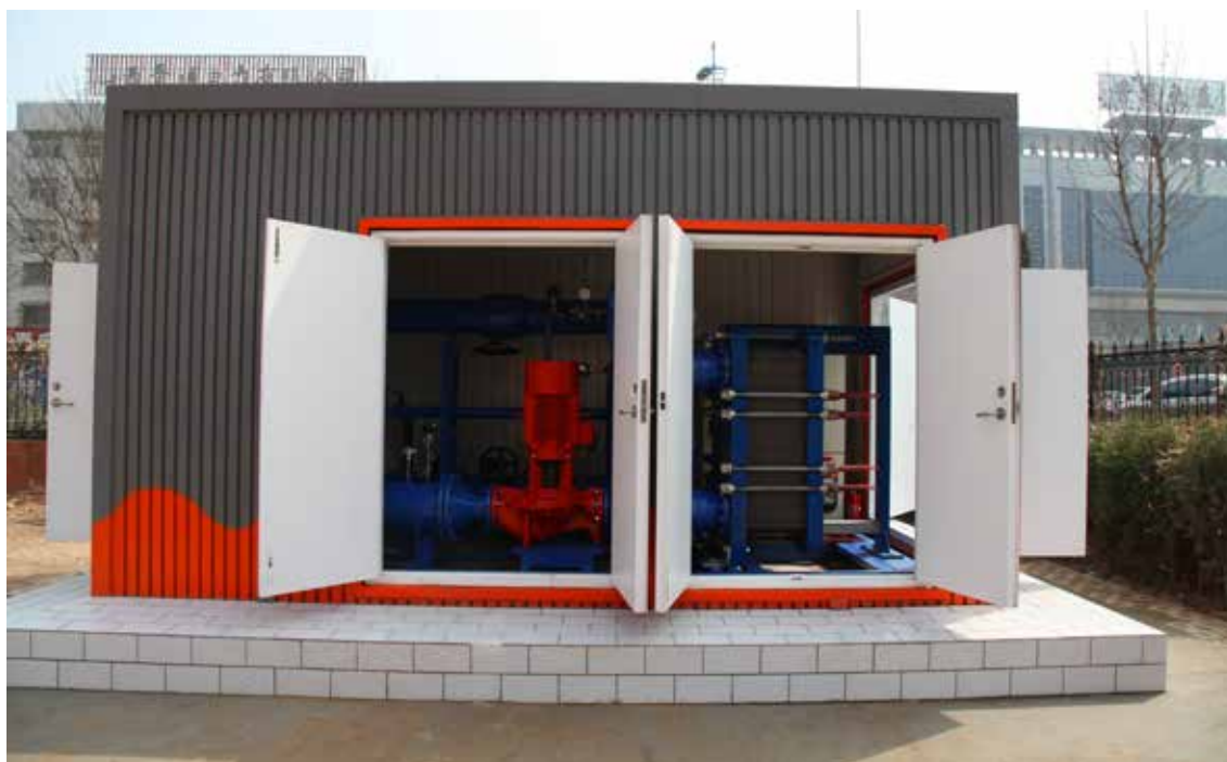
Innovative heat-exchange station with high-energy efficiency in Jinzhong 项目在晋中开发建设的高能效新型换热站
