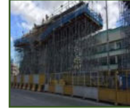
Metro Manila Skyway Stage 3
