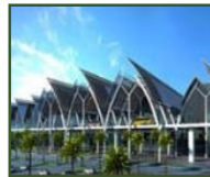
Mactan-Cebu International Airport
