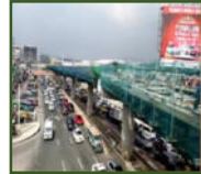
NAIA Expressway Phase (II)
