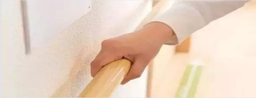
Continuous handrails in corridors and corners
