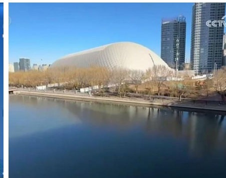
施工工地“气膜”降尘 “Air dome” for dust reduction
